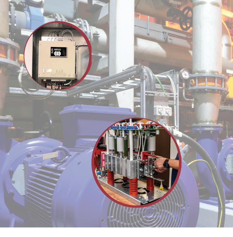
The **SI-HDN** is a heavy duty medium voltage soft starter, designed for all medium voltage AC induction motors. The **SI-HDN**'s sophisticated motor control technology ensures smooth acceleration and deceleration as it minimizes the effect of high in-rush current and mechanical torque shock.
